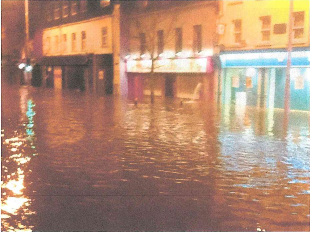
Flooding On Thomas Davis St, Blackpool , March 2013
