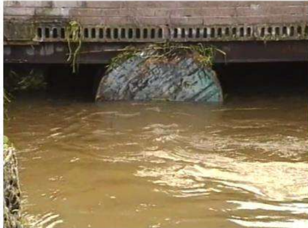
Photos 3.1 (above): Still from video of Barry Mescaill, TG4 reporting from Blackpool Bridge 2002 & Still from the video of a Telecom Eireann reel trapped under culvert entrance in 2002.
