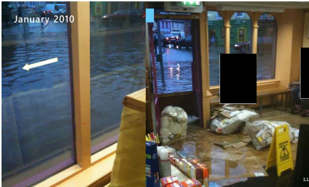
Photo 3.3: Images of flood from O'Shea's Pharmacy, Jan 2010
