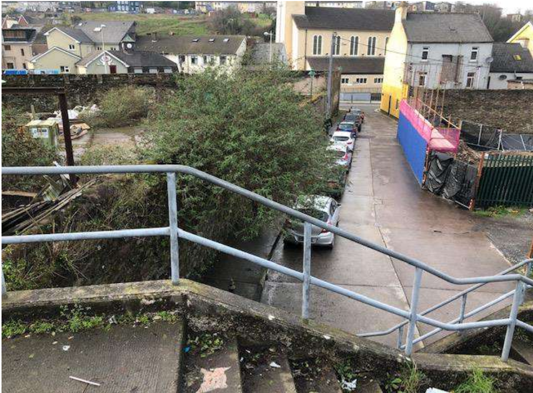
Photo 9.1: This photo taken from the Blackpool By-pass at Corcoran's quay looking west towards the church, 18/02/2020. See apartments under construction on the right-hand side at Corcoran's Quay., under the Blue tarp. Approx. 9 apartments here. Also see old OS forklift site on the left hand side of the parked cars with planning for 37 apartments, (planning notice below in Photo 9.3)
