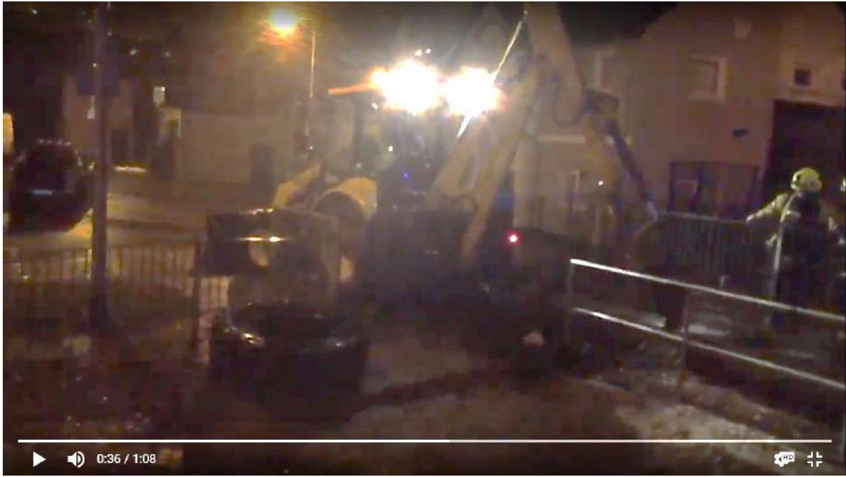
Above: Contractor removing rubbish to unblock screen in river, March 2013
