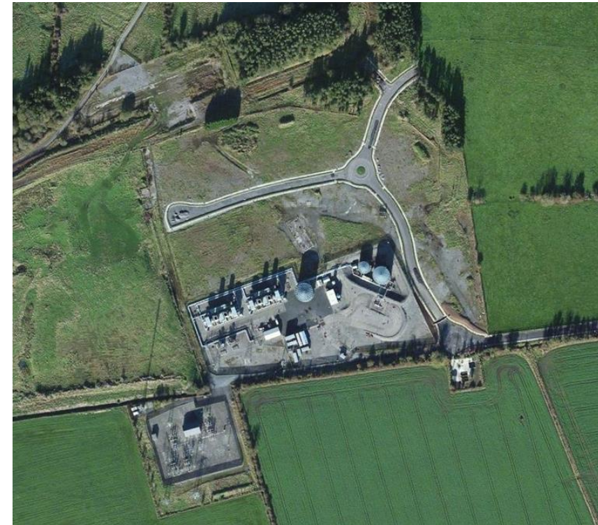
Partially complete Park infrastructure
