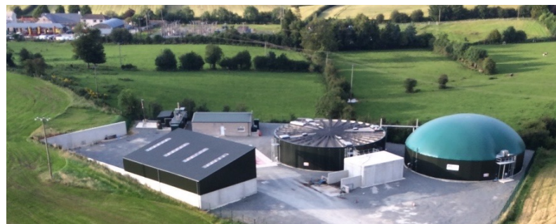
0.5MW Cookstown AD Plant
