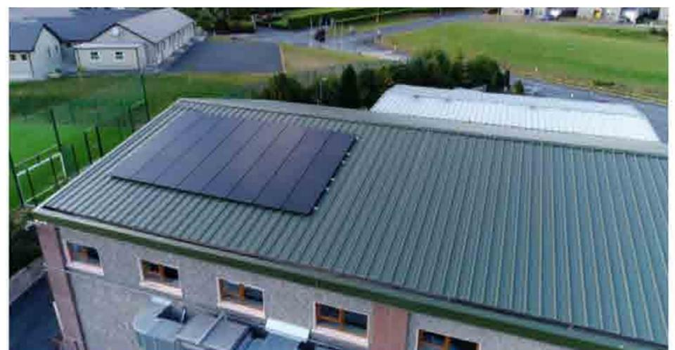
*Corduff Raferagh Community Centre roof after upgrade works and installation of solar panels.*
