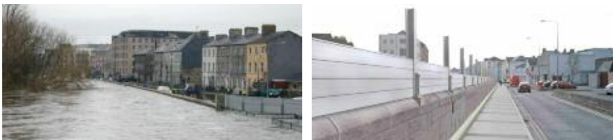
Figure 12. Flood-defence walls that kept the river water from overflowing after prolonged and heavy rainfall in 2014 (left); demountable defences which can be raised prior to potential flooding and lowered during times of low risk to reduce the visual impact on the town. A flood-warning system was developed to monitor rainfall in the catchment area to make sure the defences are fully installed before a flood (right) (McCarthy, 2015; Mott MacDonald Ireland).
