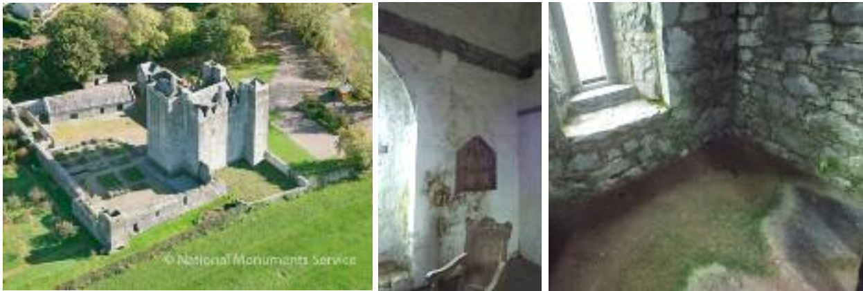
Figure 25. Aerial view of Barryscourt Castle, County Cork (left) (DCHG); mould growth on the interior of the castle (centre and right) (OPW)
