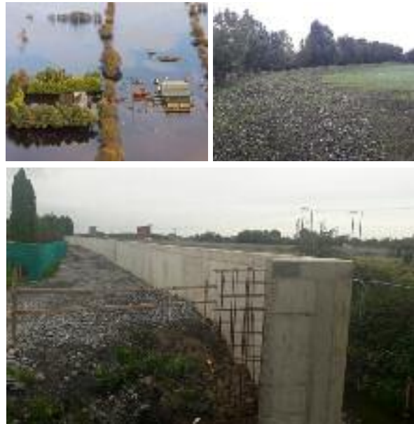
Figure 14. Flooding near Athlone town along the River Shannon (left) (Fitzsimons, 2018); implementation of a flood embankment (right) and flood-defence wall (below) on Brick Island in Athlone (Athlone Flood Alleviation Scheme Project Team, 2019)
