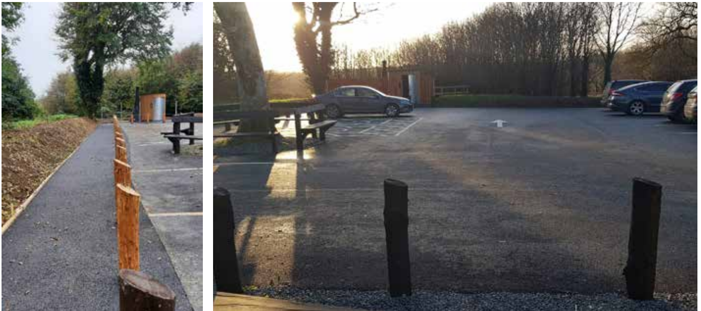
Tintern car park with dry toilet and safe access route to same.
