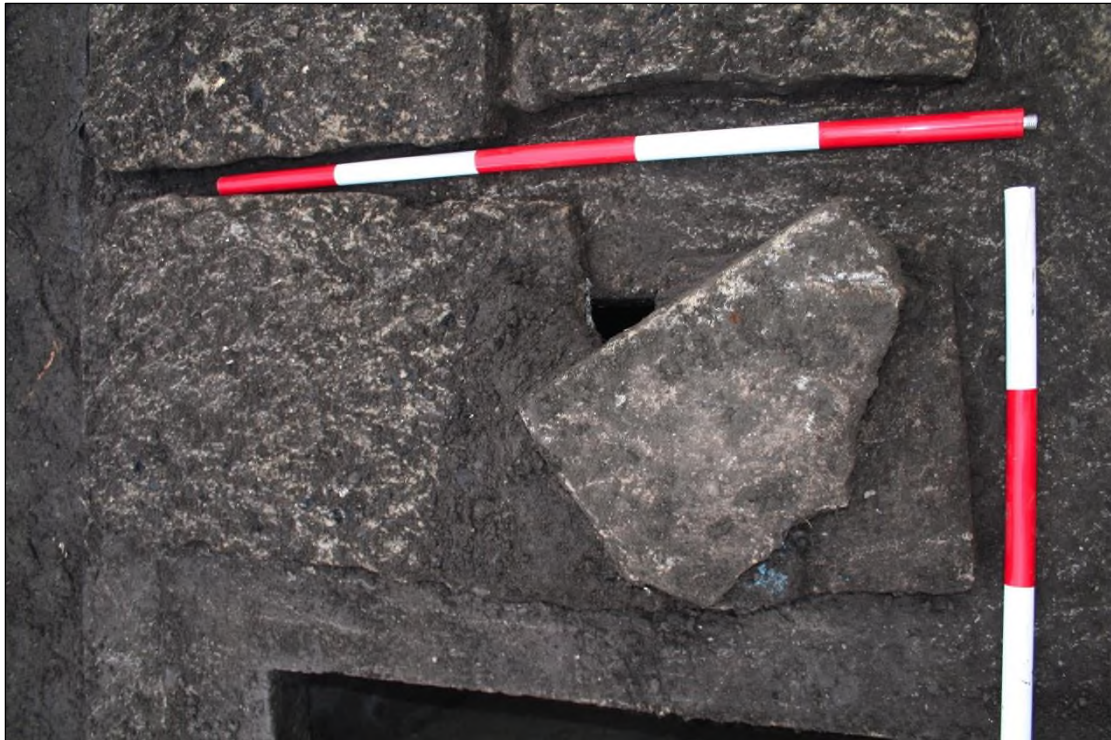
Plate 2.6: Evidence of damage to original lids.
