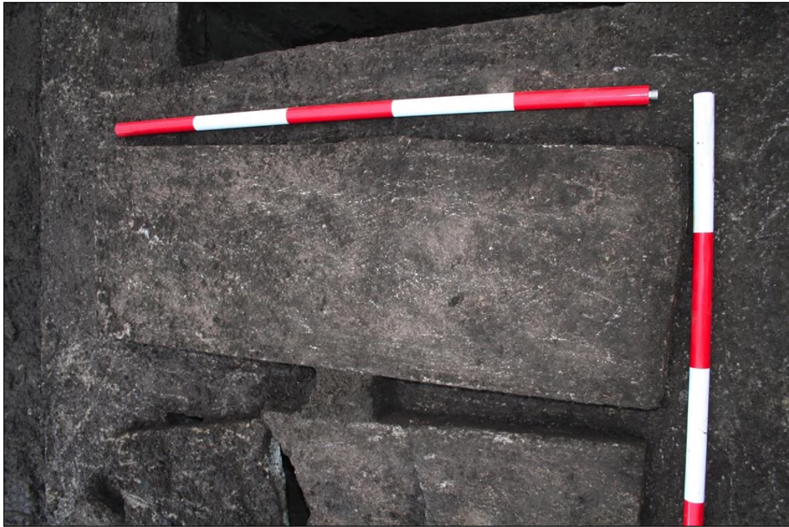
Plate 2.4: Concrete lid consistent with original concrete structure
