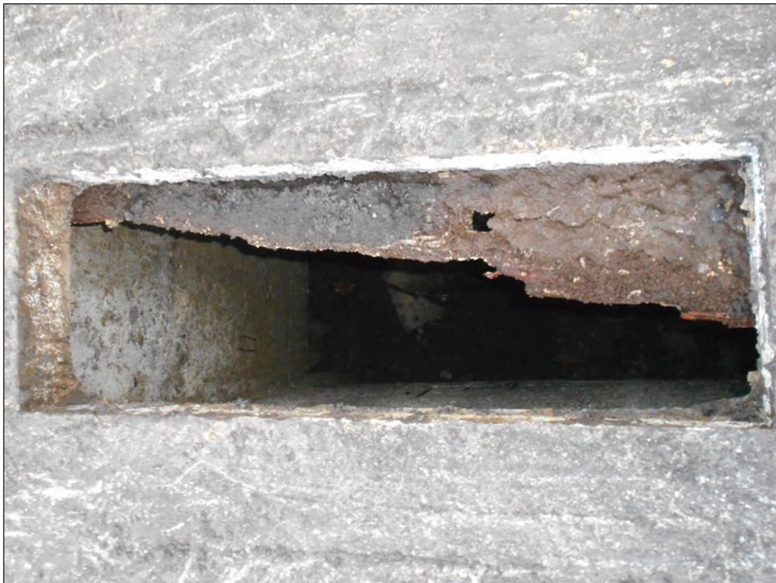
Plate 2.3: Timber formwork in situ at C.46/47/62/63
