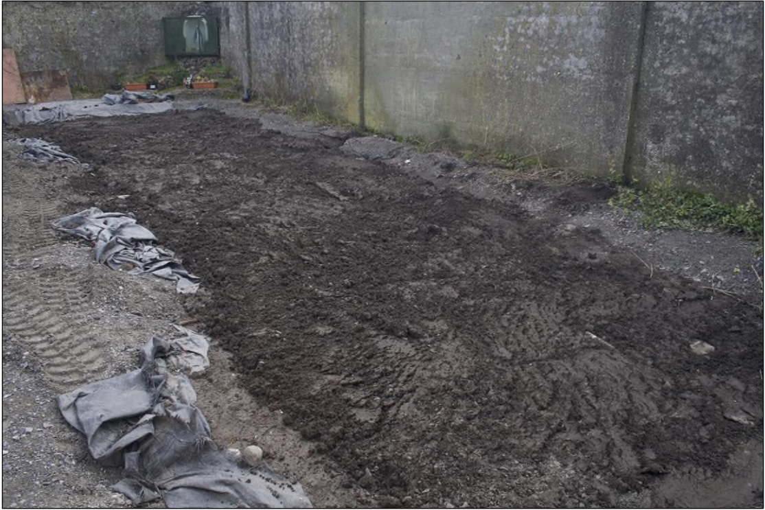
Plates 6.3: Overburden reinstated
