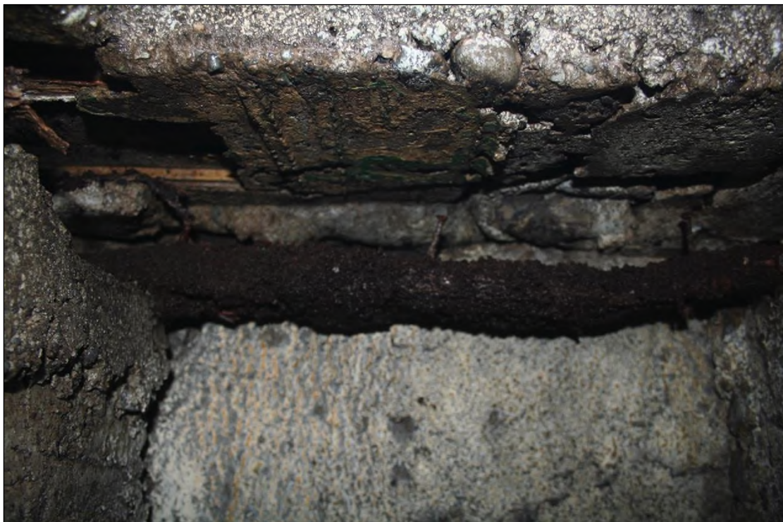
Plate 2.7: Timber in situ for cast concrete cap (C.5) at C.73/74/92/93
