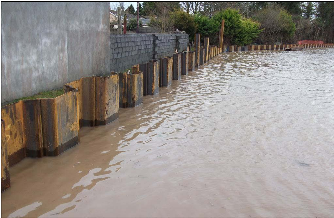
February Flooding during construction
