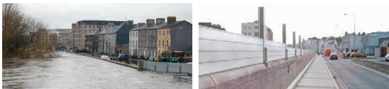
Figure 12. Flood-defence walls that kept the river water from overflowing after prolonged and heavy rainfall in 2014 (left); demountable defences which can be raised prior to potential flooding and lowered during times of low risk to reduce the visual impact on the town. A flood-warning system was developed to monitor rainfall in the catchment area to make sure the defences are fully installed before a flood (right) (McCarthy, 2015; Mott MacDonald Ireland).
