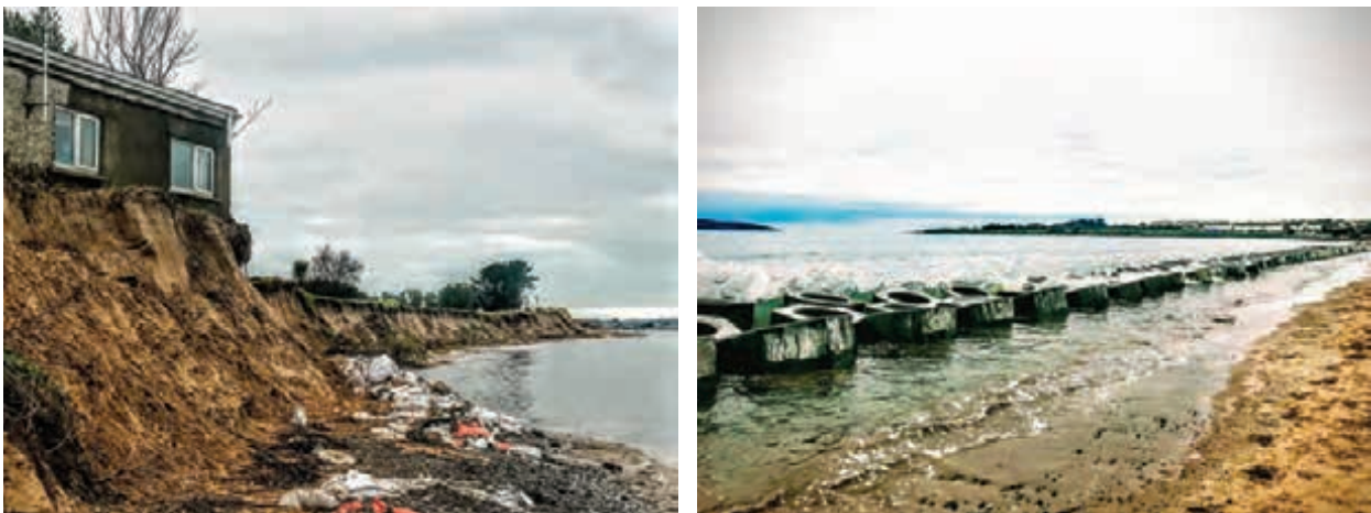
Figure 9. Dwellings in Portraine on the brink of falling into the sea because of coastal erosion (left); €500,000 worth of concrete blocks installed as a short-term solution to coastal erosion in Portraine (right) (Comerford, 2018)
