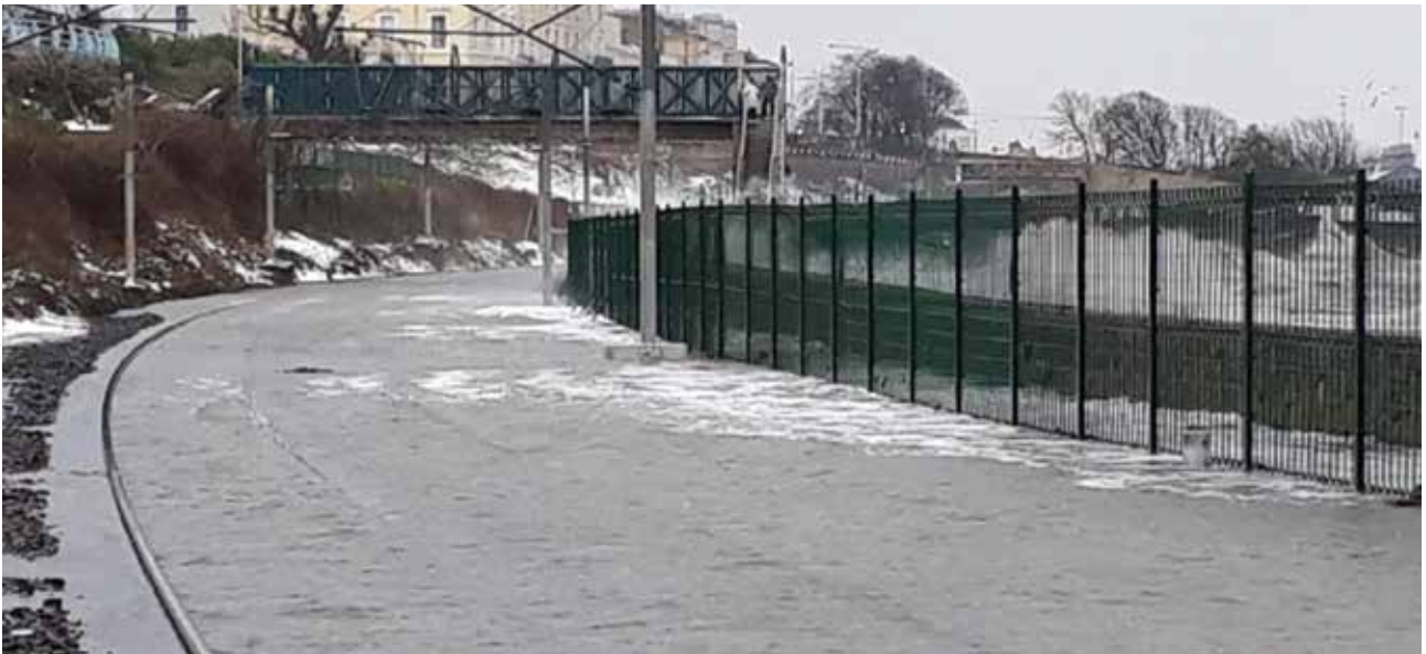
Figure 3.13 Tidal surge flooding exacerbated by SLR at Salthill and Monkstown DART station in Dún Laoghaire-Rathdown, Co. Dublin, February 2018. Source: Irish Rail.
