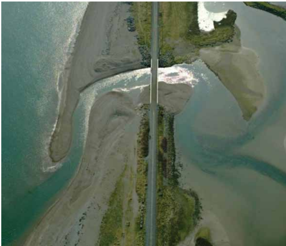
Figure 3.14: The Eastern rail line is subject to erosion as it traverses the Breaches River at Kilcoole, Co. Wicklow. Source: ÍarnródÉireann LIDAR Study, 2011.
