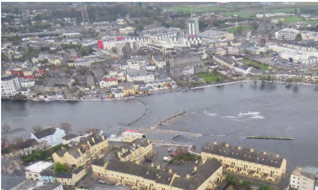
Figure 3-3: Flooding of the River Shannon at Athlone
