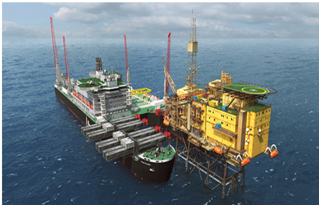
Figure C3 - Removal of platform topsides in single lift (option using specialist HLV – courtesy of Allseas)
