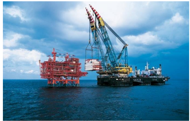
Figure C2 - Removal of platform topsides using multiple lifts (option using conventional heavy lift vessel (HLV) – courtesy of Saipem)
