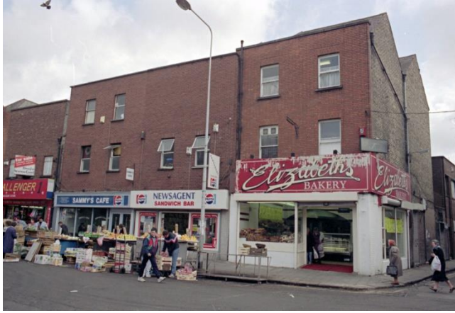
Fig 3: No 10 Moore Street 1991 showing Moore Lane brick gable removed and replaced by a full shop window.
