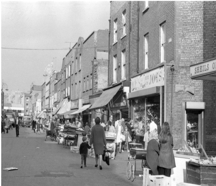
Fig 2: Moore St 1971 showing sealed up gable of No 10 in right foreground.
