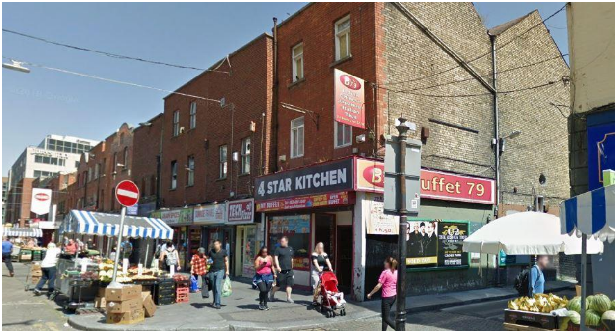
Fig 4: Gable end No 10, 2018
