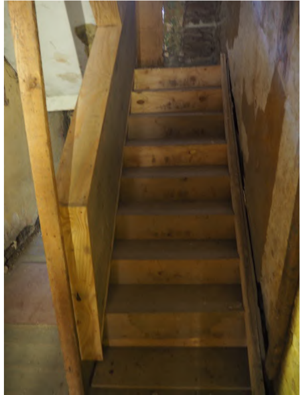
P16.2 Protection in place on a staircase
