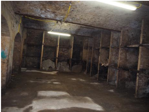
P43.4 The sub-terranean cellars at 8 and 9 Moore lane
