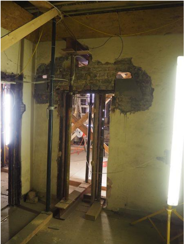
P15.3 One of the new openings to allow circulation between buildings
