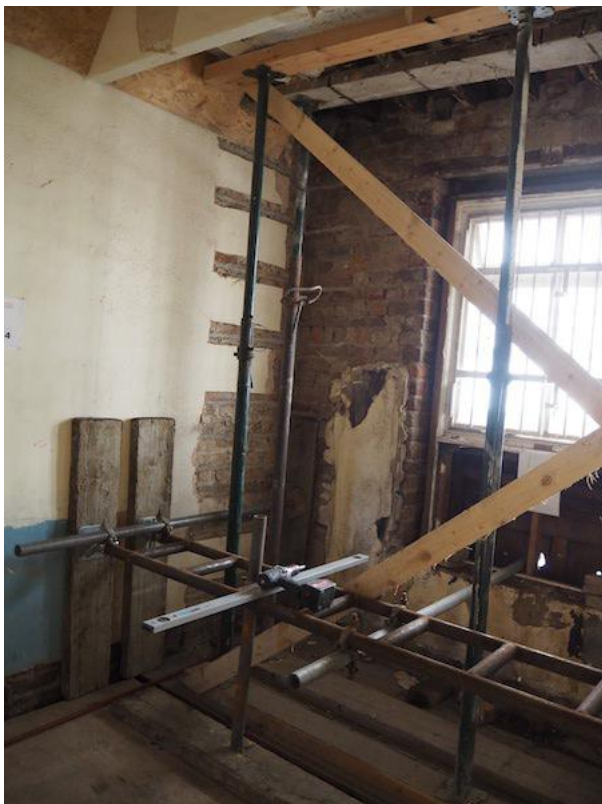
P28.3 Some of the propping and restraint systems are quite elaborate
