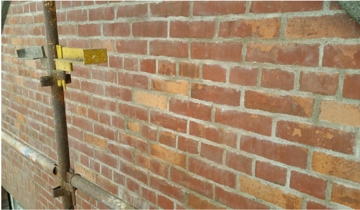
Example of temporary pointing on parapets (Photo: P. Walsh)
