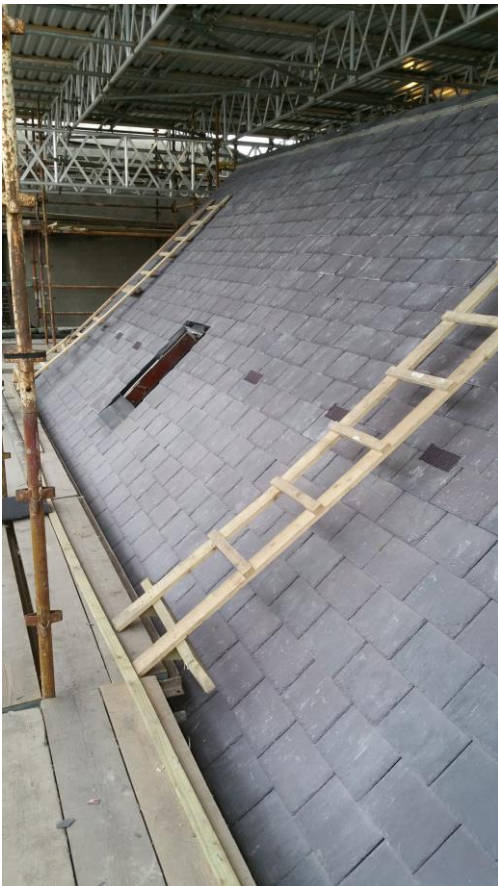
Slating on roof of no. 17 (Photo: P. Walsh)
