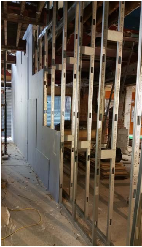
Fire-proof partition between nos.17A/18 (Photo: P. Walsh)
