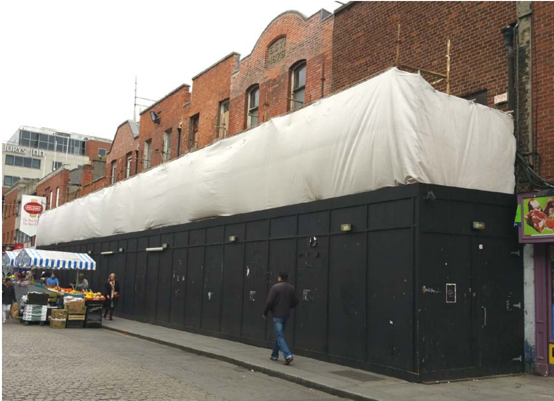
Buildings reappearing as the scaffolding is being reduced (Photo: P. Walsh)
