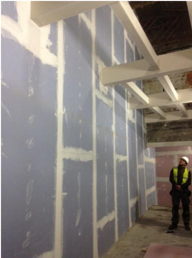
Fire-proof partition on site perimeter (17A) (Photo: A. Lynch)
