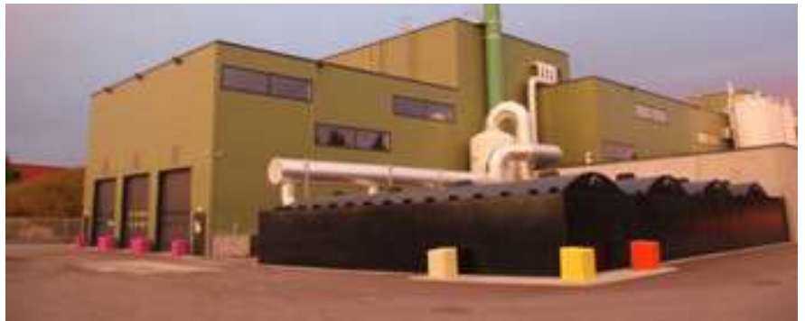
Image: Biogas plant (City of Oslo)
