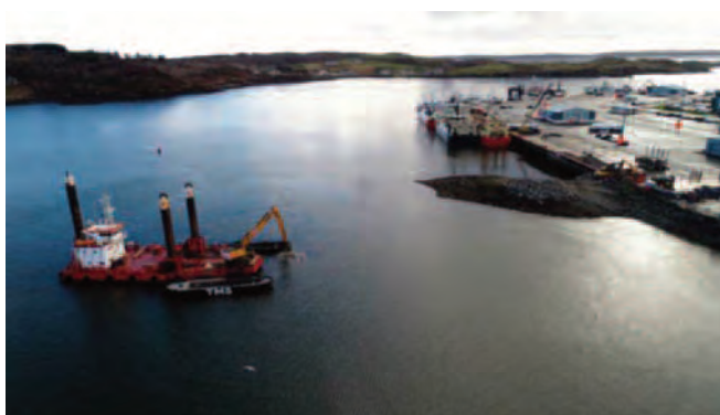
Smooth Point Quay Extension, Killybegs FHC Dredging Works in progress 2019
